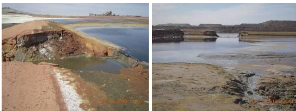
Figs. 43-44 Spill of contaminated slurry at Somair-AREVA Mine, Niger
