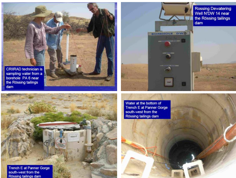
Figs. 27-30 Dewatering wells and trenches designed to pump back contaminated water to the Rössing tailings dam, Namibia
